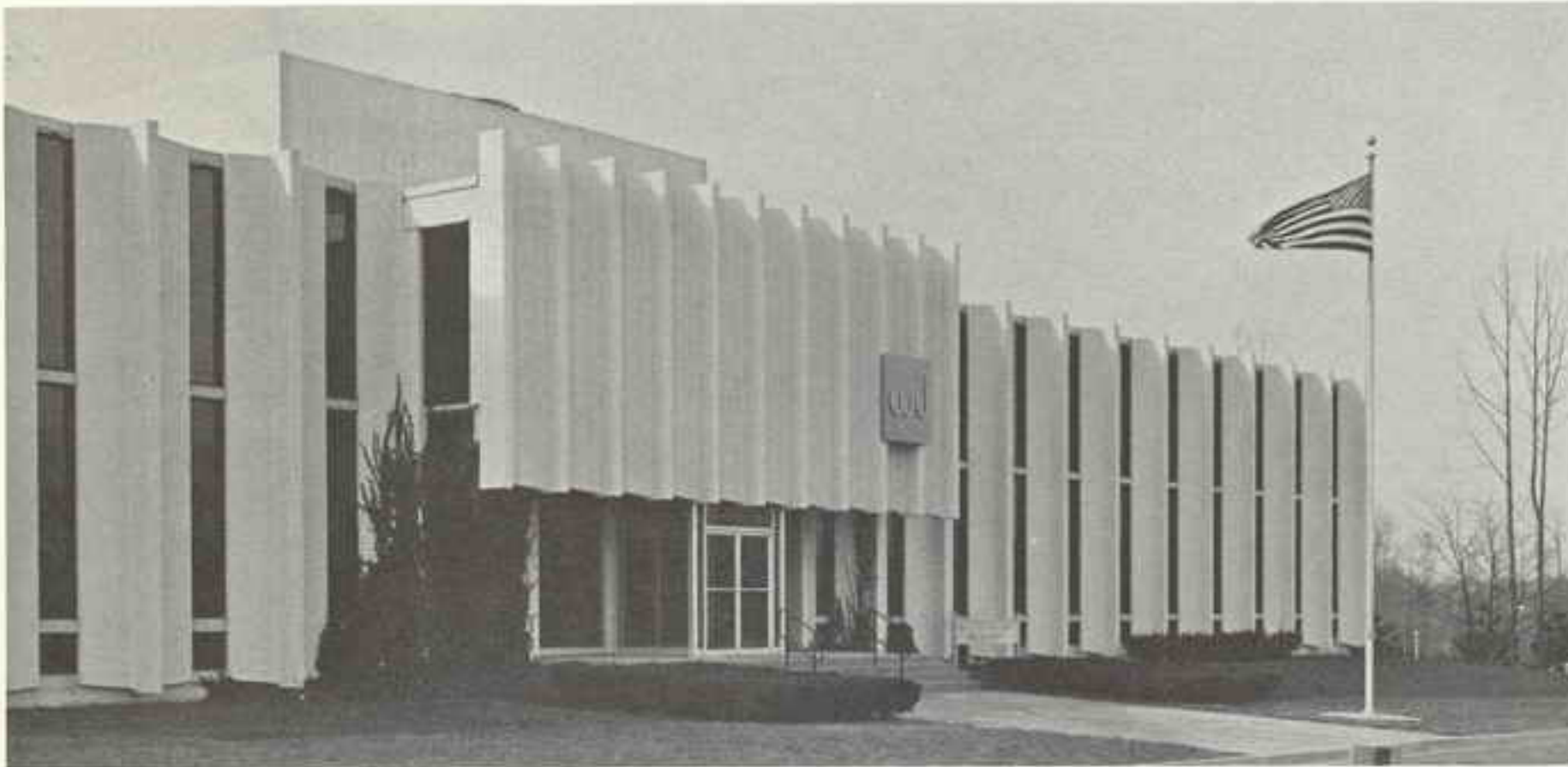
Watkins-Johnson - Rockville facility
